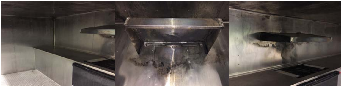
Walls and kitchen hood
